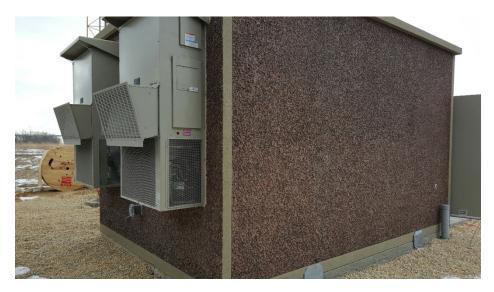
• Rear exterior view of the Brigham shelter. The two large, tan boxes on the left are the HVAC units. Both are identical and able to support the HVAC needs of the shelter individually. Two are installed at each shelter to provide backup / redundancy should one unit break down.
