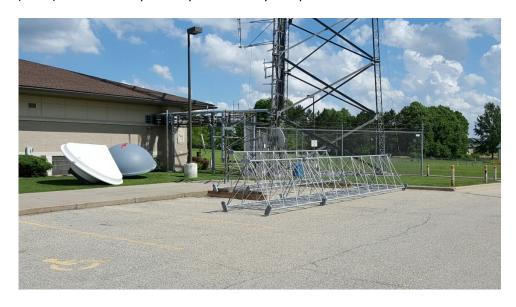
• Close-up photo of a radio tower section (this one at DeForest before it was installed above)
